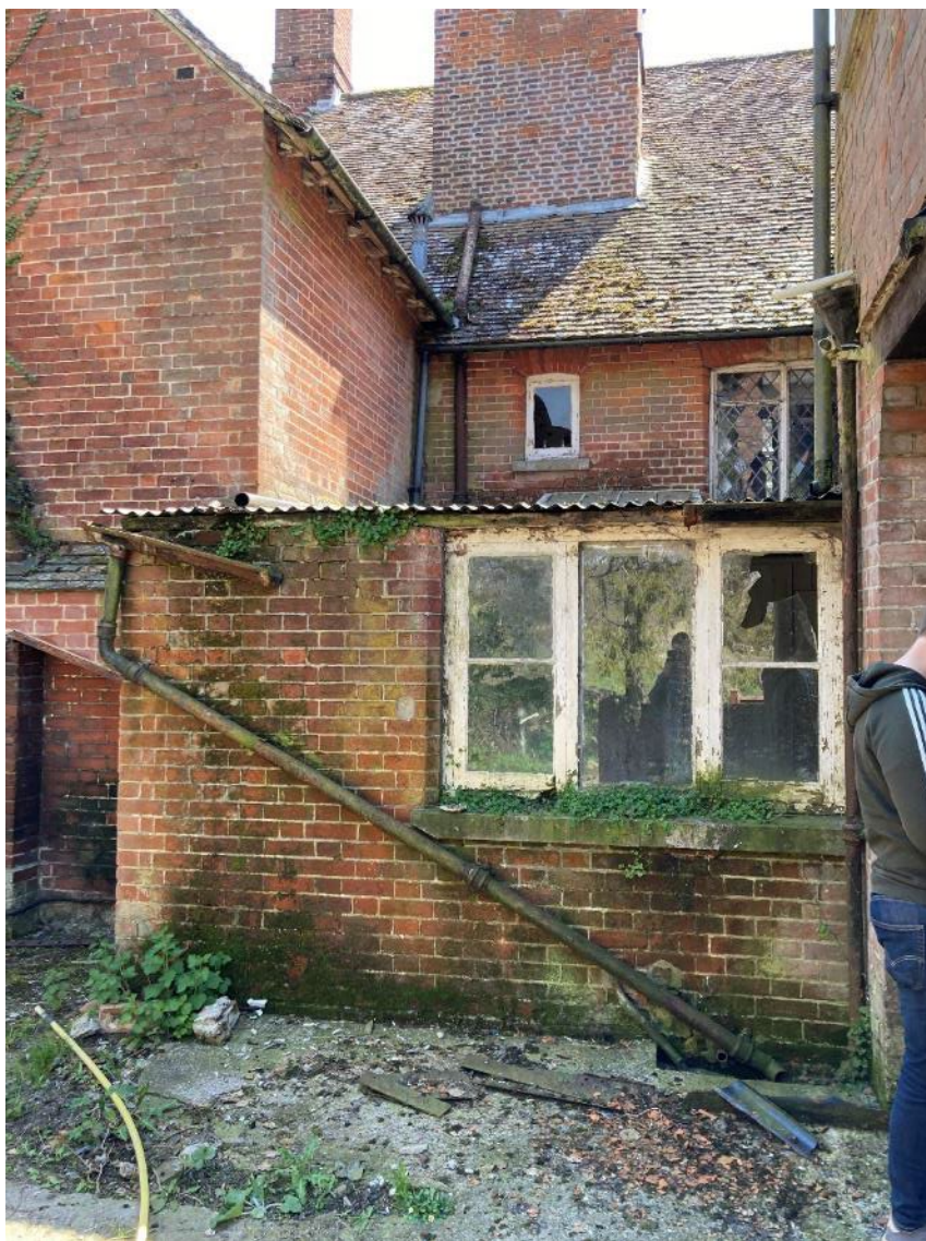
Plate 11: View of rear central extension
