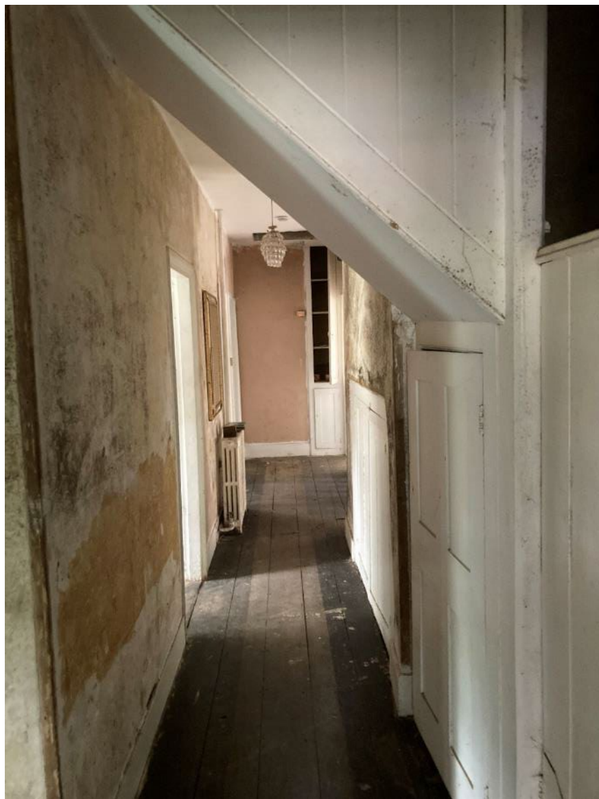
Plate 19: First floor landing
