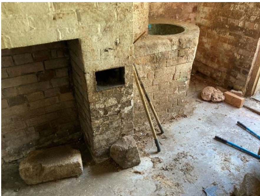
Plate 38: Room 7 showing wash room area
