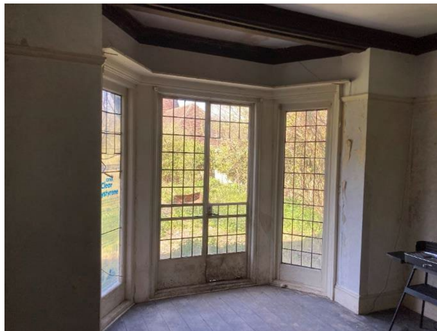
Plate 31: Room 8 showing bay area below modern extension
