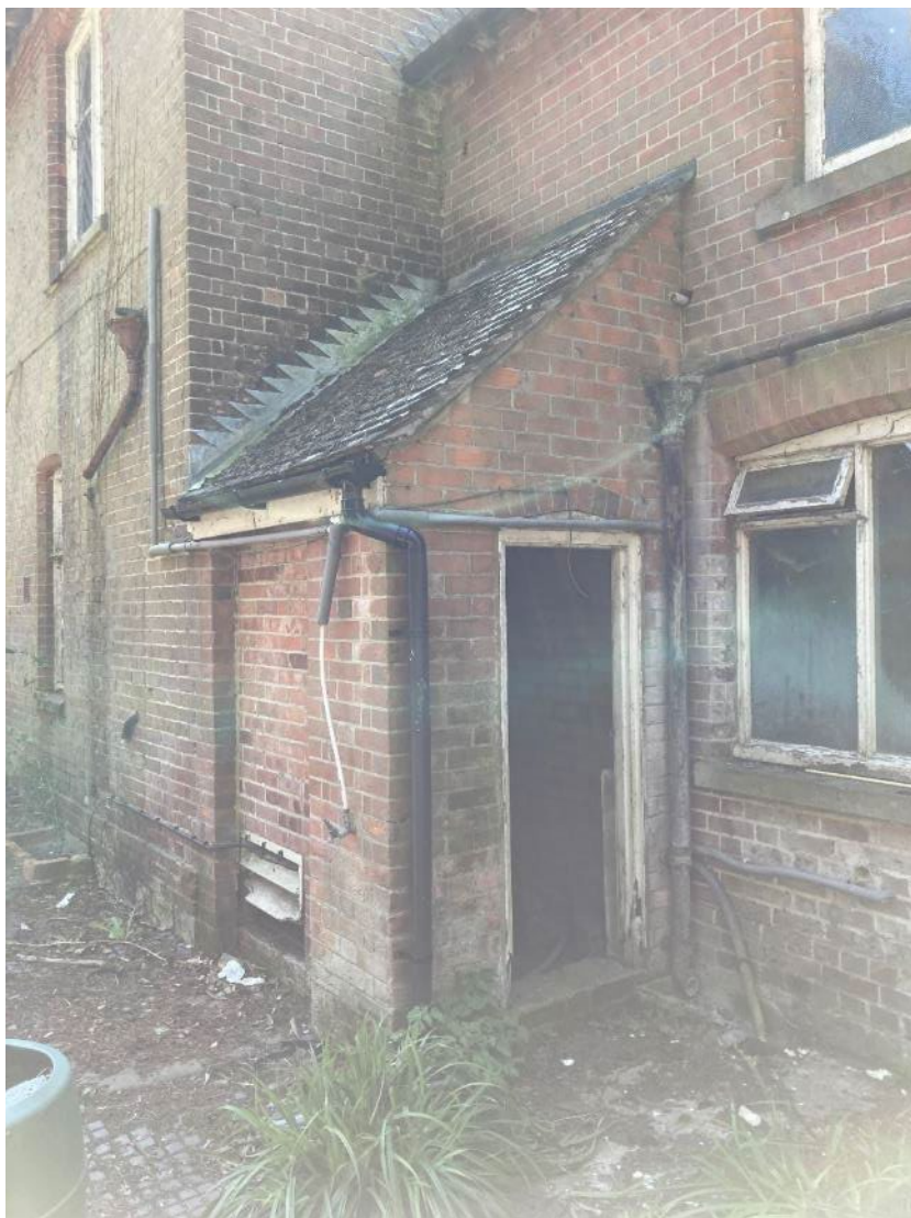
Plate 9: View of small extension on eastern elevation
