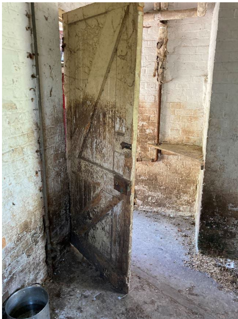
Plate 36: Room 7, showing part of wall area to be demolished
