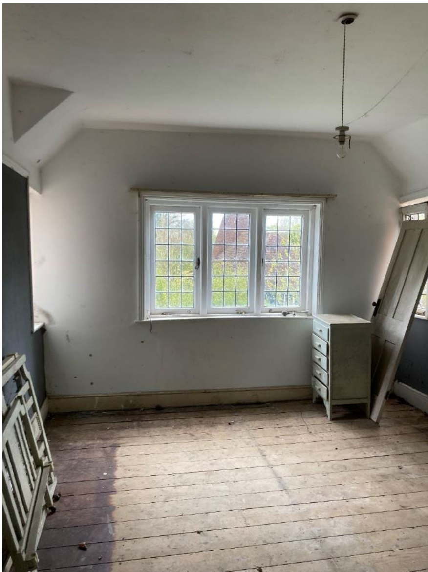
Plate 30: Room 4, showing modern extended area
