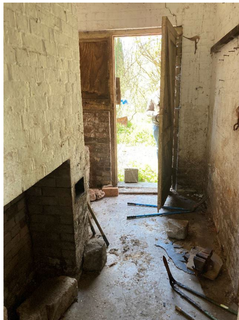
Plate 37: Room 7, showing part of wall area to be demolished
