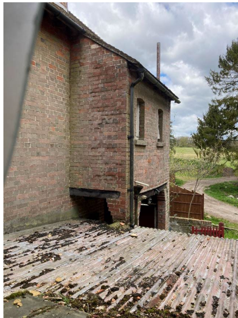
Plate 16: View to the rear of the western wing
