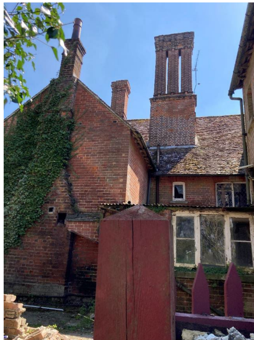
Plate 12: north easter rear extension area
