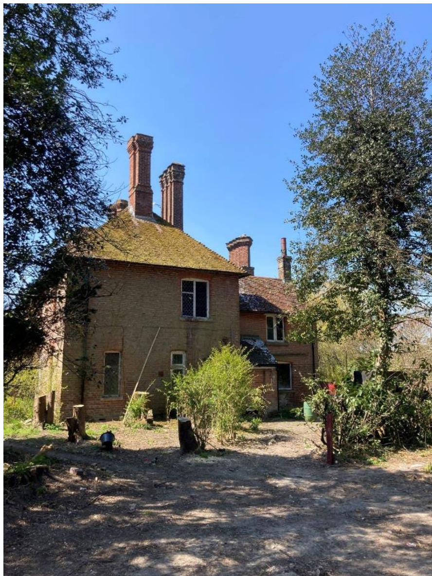
Plate 8: View of eastern elevation
