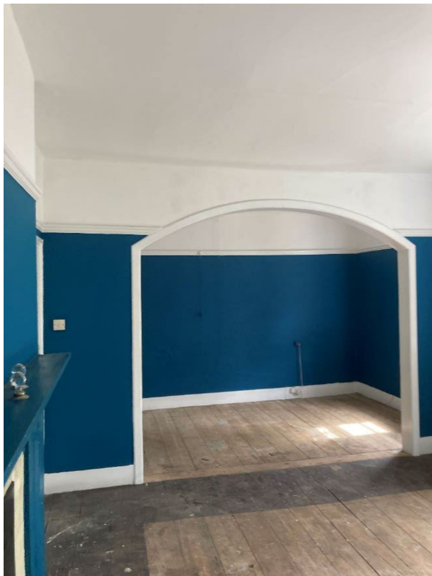
Plate 17: Room 10, Existing opening to remain
