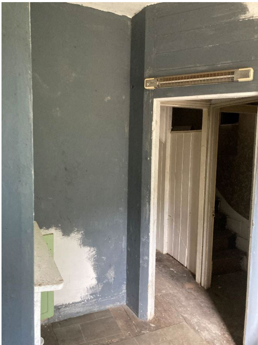
Plate 23: Room 2, showing area to be knocked through
